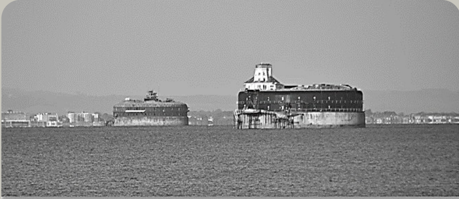
No Man's Land and Horse Sand forts flanking the main shipping channel
